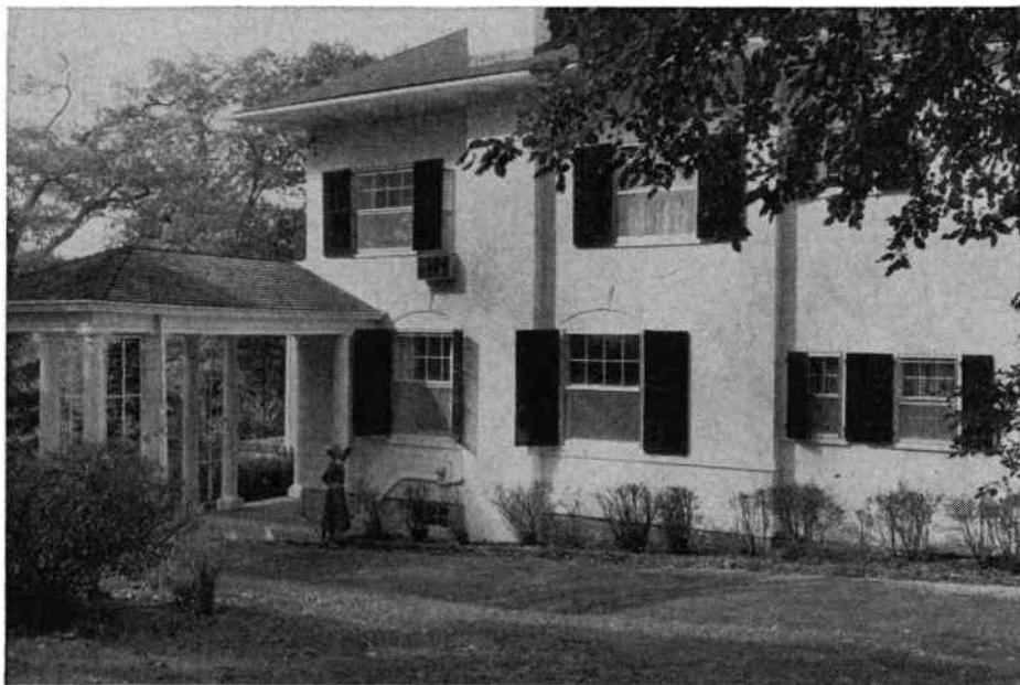
FOR PRIVACY, Betsy and her husband purchased this twelve-room house in Englewood, N. J., last April, are remodeling it. Betsy was architect, decorator.
